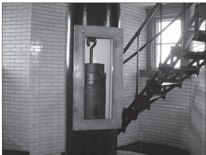
Weights visible in drop tube window, originally an access door. Split Rock, Minnesota. Photo by the author.
