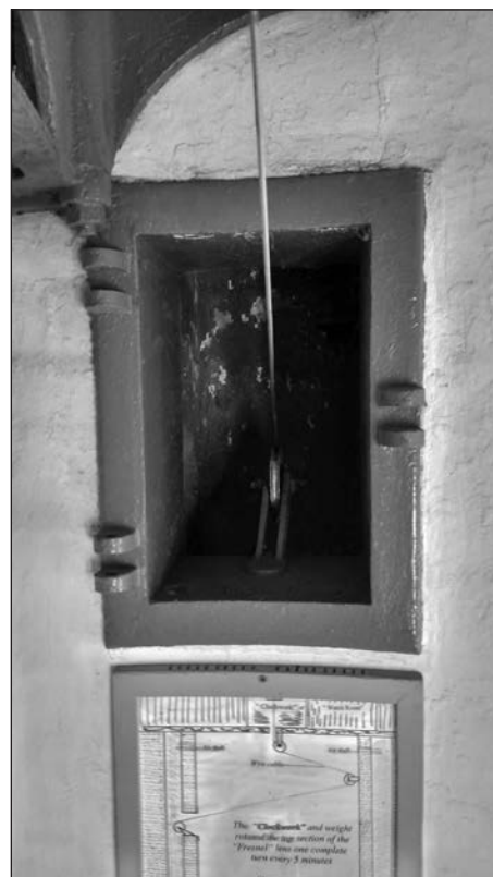
Upper door opening into inner-wall space (door removed), showing cable going around the pulley inside. Little Sable Point, Michigan. Photo by Matt Varnum, SPLKA.
