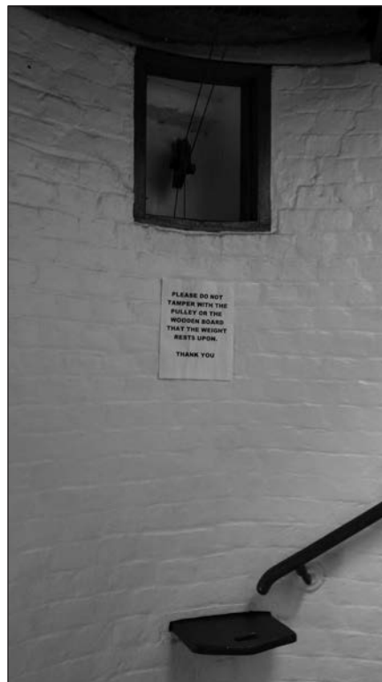
Photo shows both the upper access door and the weight-resting shelf below. White River, Michigan. Photo by Matt Varnum, SPLKA.
