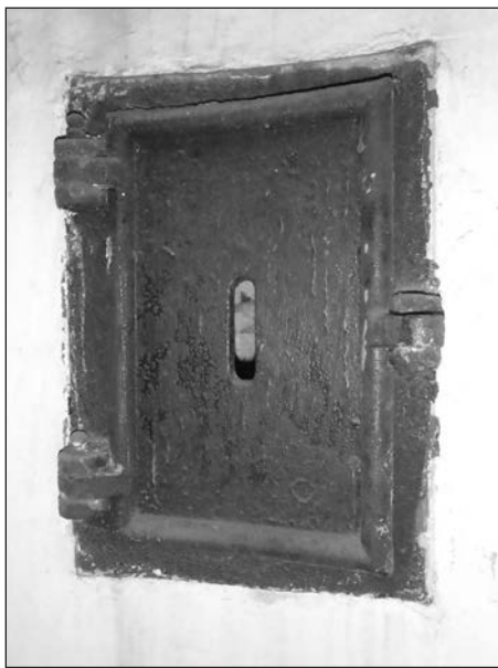
Upper doors into inter-wall space at (above) Cana Island, Wisconsin (photo by Lee Radzak) and (below) Outer Island, Wisconsin (National Park Service photo by David Cooper.)
