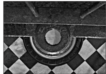
Below: Guide “eye” on landing for the weight cable, centered over the weight pit at St. Augustine. Photos by Kathleen McCormick.
