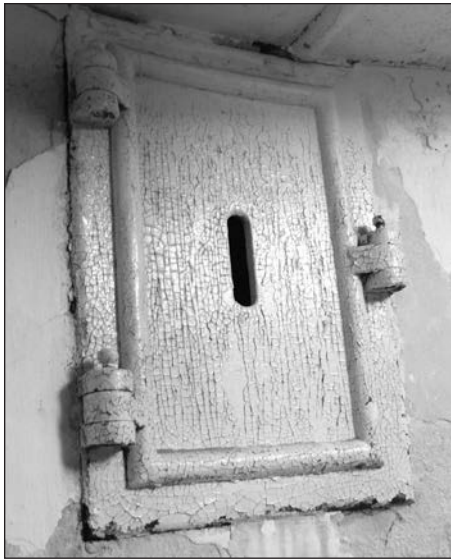
Upper doors into inter-wall space at (above) Cana Island, Wisconsin (photo by Lee Radzak) and (below) Outer Island, Wisconsin (National Park Service photo by David Cooper.)
