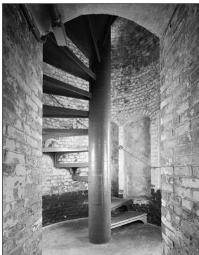
Central stair column that also serves as weight tube, Burnt Island, Maine. U.S. Coast Guard photo.
