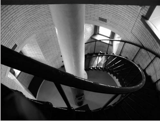
Centered drop tube, Split Rock, Minnesota. Photo by Lee Radzak.
