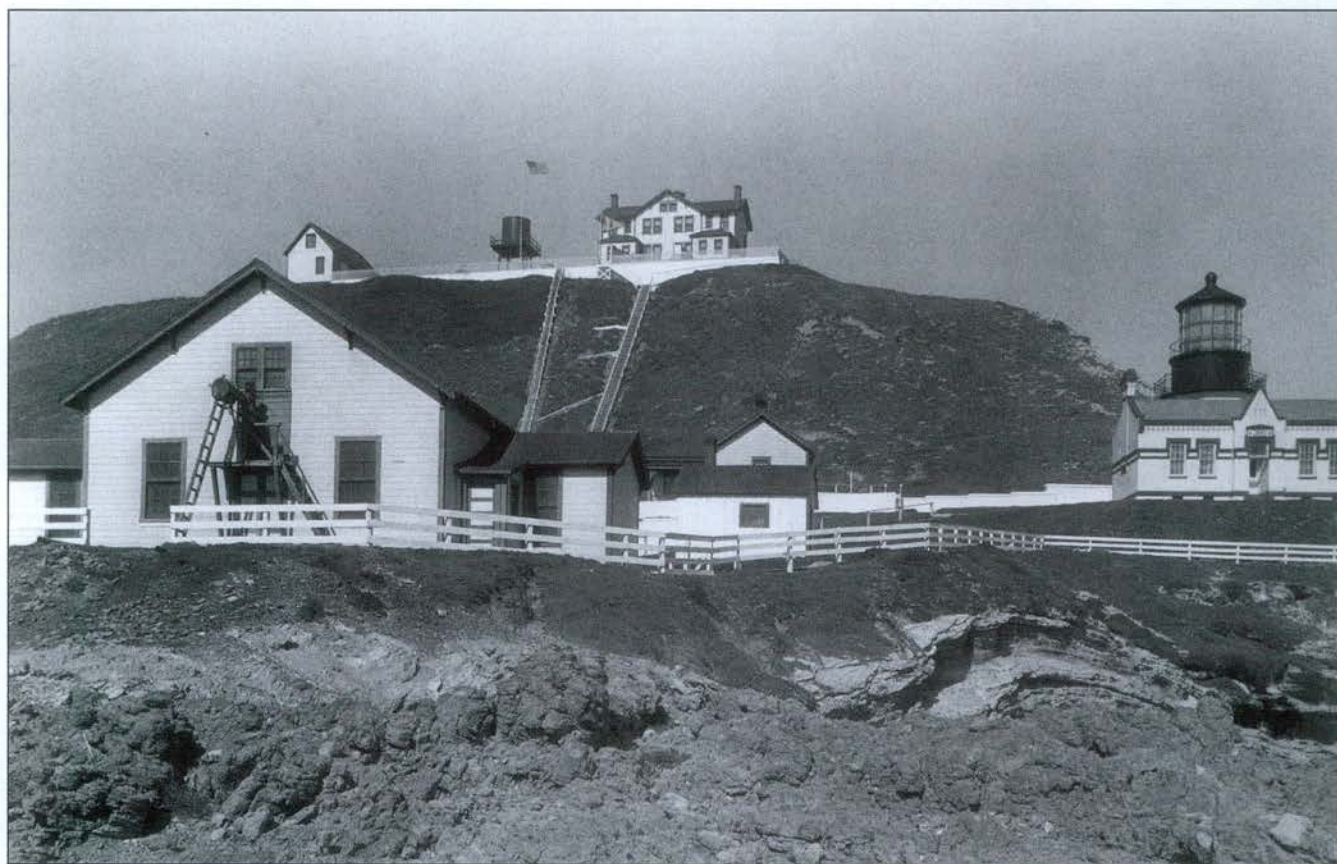
Fog signal at left, 3rd assistant keeper house center, lighthouse right. The left ribbon descending the hill is the supply chute used to send coal, and other supplies, down to the fog signal building and assistant's dwelling.
