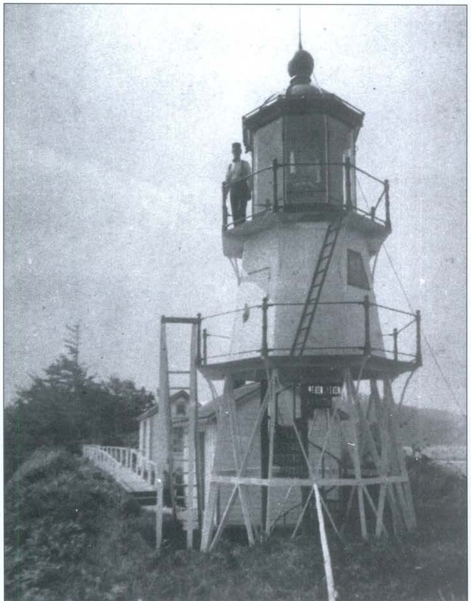
The first Cape Arago Lighthouse constructed in 1866. The small structure under the tower is probably a watch room and the structure behind it, a storage shed. The keeper appears to be wearing a uniform hat, which dates the photo between 1884 and 1896. USLHS photo.
