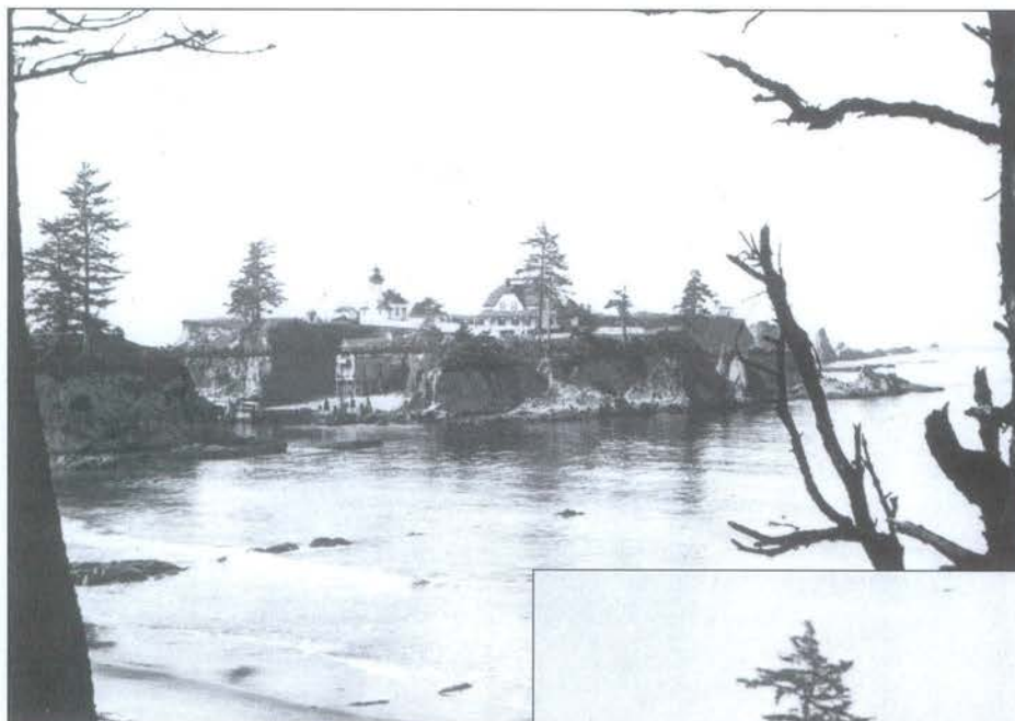
Left – A view of the Cape Arago station from the north with open sea to the right. Note the stiff legged crane and Life Saving Service building in the cove. The 1st (abandoned) light tower can barely be seen at right alongside the 1898 fog signal building.
