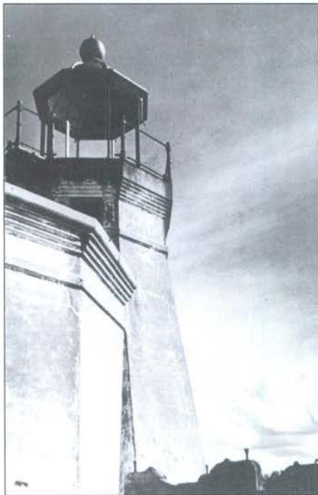
The original 1866 Cape Arago tower (encased in brick in 1896) shortly before it was blown up in 1936. Oregon Journal photo.
