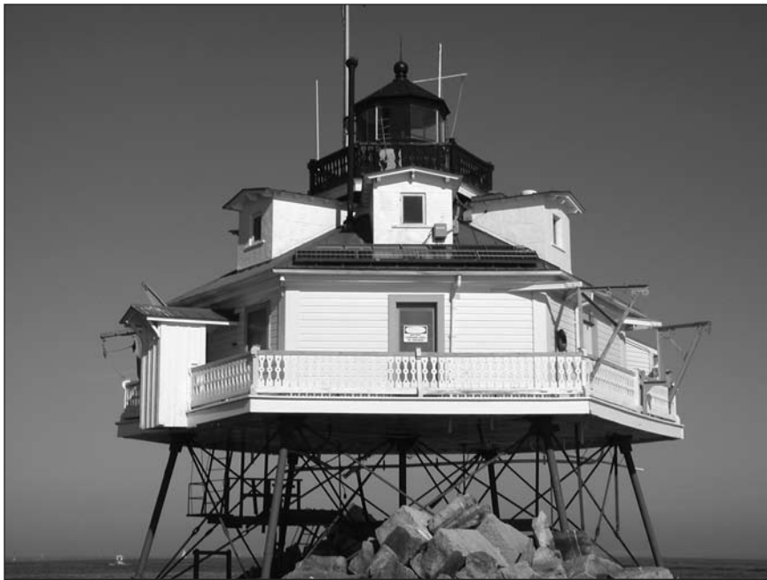
Above left – The original privy, with direct drop into the bay can be seen at left. At right is one of the davits to hoist the station boat up to deck level. Above right – The interior of the privy indicating that the pigeon had a difficult time hitting the hole.
