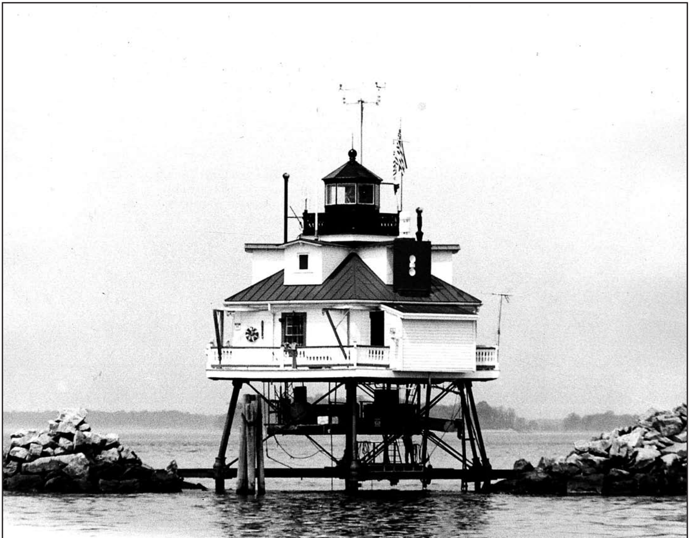
Thomas Point Shoal Lighthouse in recent years when manned. Rock piles on the up-bay and down-bay sides are to divert ice floes. Above the storage shed, at right on the main deck is the electronic, pure-tone sound (fog) signal. Photo by Joan Mullaney.
