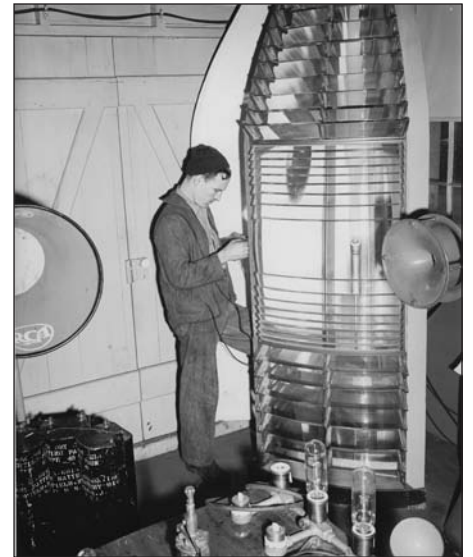
U.S. Coast Guard lampist assembles a lens, circa early 1960s. U.S. Coast Guard photo.
