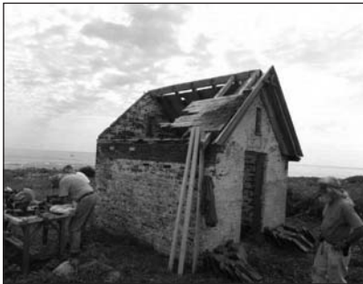
Before (above) and after (below) photos of the oil house. Thacher volunteers completely restored this oil house adding a new roof, trim, door, copper flashing, and lightning arrestors.
