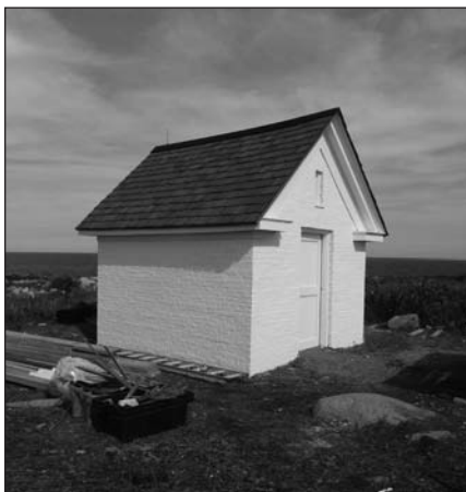
Before (above) and after (below) photos of the oil house. Thacher volunteers completely restored this oil house adding a new roof, trim, door, copper flashing, and lightning arrestors.
