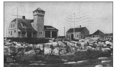
Gap Cove Life-Saving Station.
