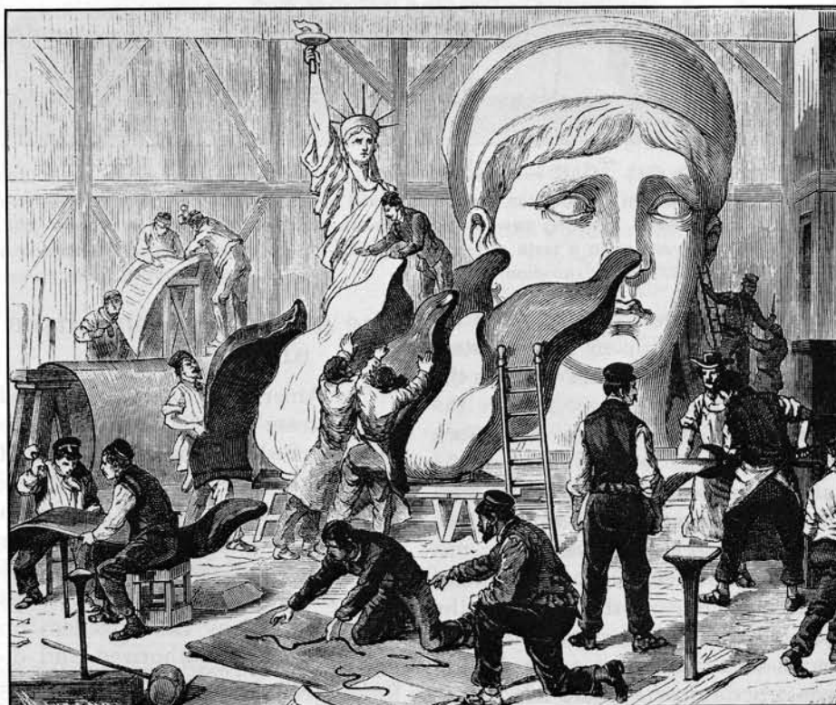
Bartholdi’s creation blossomed forth from flat sheets of copper tediously worked. The head and right hand clutching its torch were the first features to be completed in their mammoth proportions.
