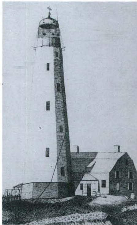
Sandy Hook Lighthouse in 1790 by I. Anderson, engraved by Cornelius Tiebout. There appears to be wire mesh around the lantern room. It might have been installed to prevent birds from smashing the storm panes at night.
