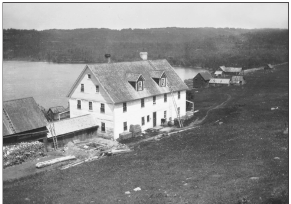
The buildings used as a residence and office for engineer Tinkham and his crew are at far right. The large building in the foreground is a private men's hunting and fishing club, and formerly the offices of a copper mining company. Photo courtesy of Isle Royale National Park.
