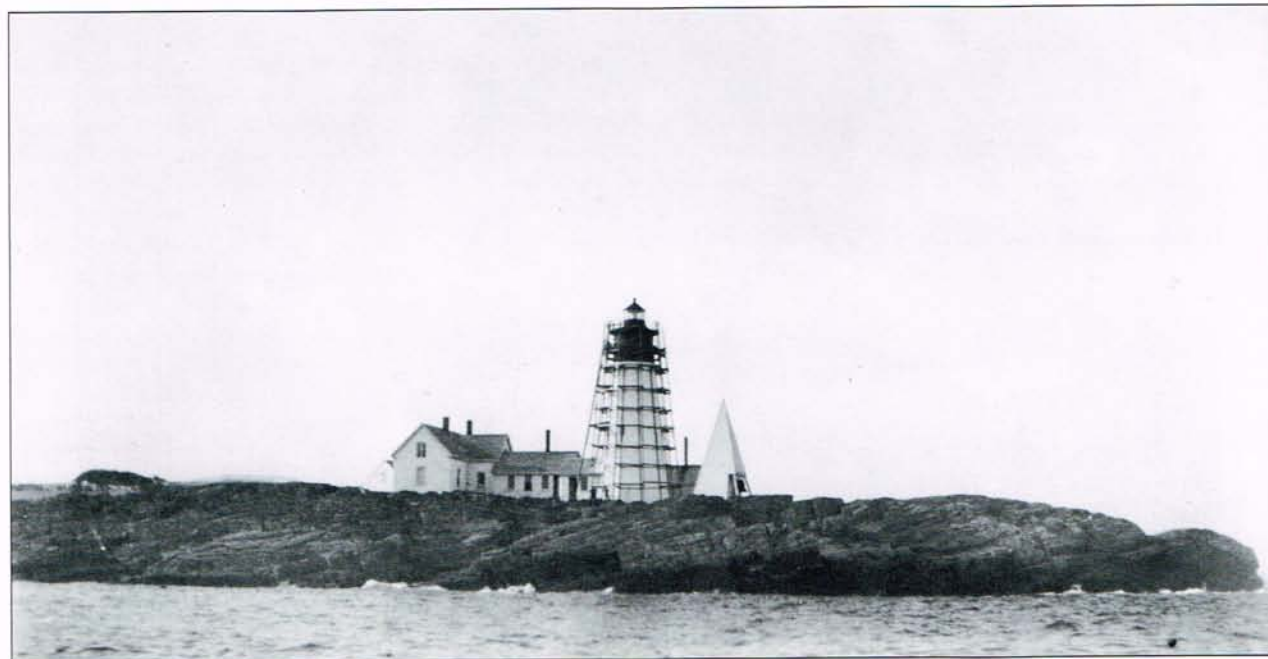
In the latter part of 1884, this scaffolding was erected to raise the height of the tower 20 feet, the height which it had been just one year earlier. During the time when the tower was at the lower level, mariners complained that they could not distinguish the light from those on ship masts or shore lights. Photo courtesy of the Maine Historic Preservation Commission.
