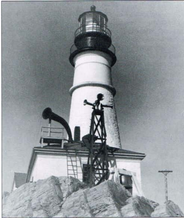
In 1938 a three horn Diaphragm Chime Horn finally replaced the Daboll trumpet (seen at left). The center and largest horn, of the new system, pointed to the Halfway Rock lighthouse. The two smaller horns were directed to the Portland Lightship and the harbor. Note the old bell mounted at right. National Archives photo.
