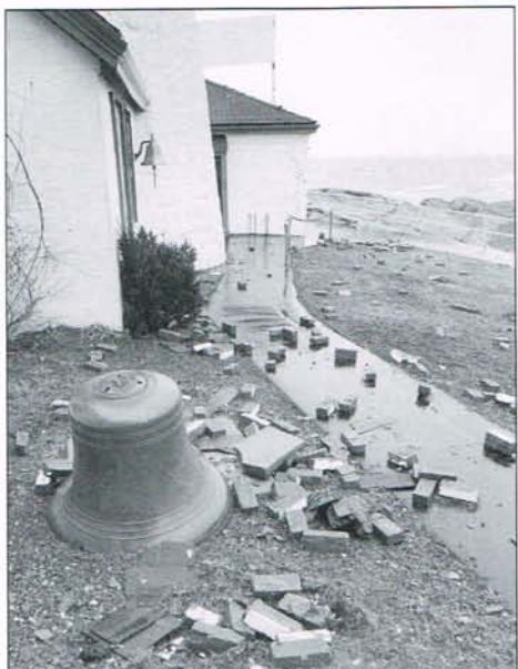
Right - The power of the sea is all too evident in this old photo of a storm at Portland Head. Above - Cracks in the brick work can be seen on the right side of the fog signal building (structure at right). The bell stand that held the 1,200 lb. bell (in the foreground) was completely destroyed. Photo by Charles Merrill, courtesy of the Evening Express.
