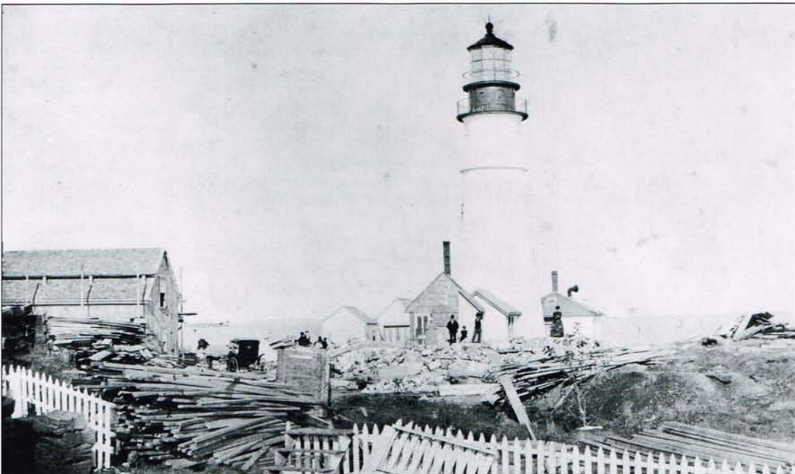
This 1890 photo shows the remains of the demolished keeper's house and piles of lumber which were used in the construction of the present elegant double dwelling. Photo courtesy of the Cape Elizabeth Historical Society.
