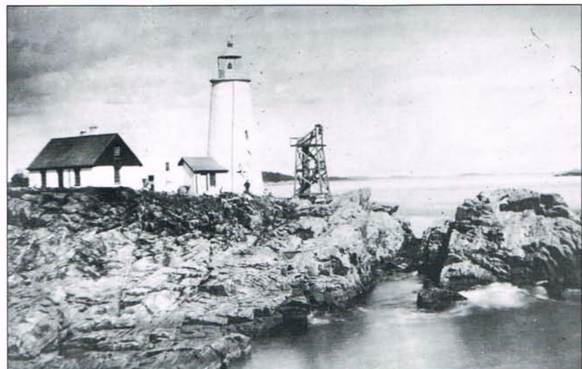
One of the earliest known photographs of Portland Head (circa 1858) shows the tower and keeper's dwelling as originally constructed, and the 4th order lens and bell tower which were established in 1855. Photo courtesy Maine Historic Preservation Commission.
