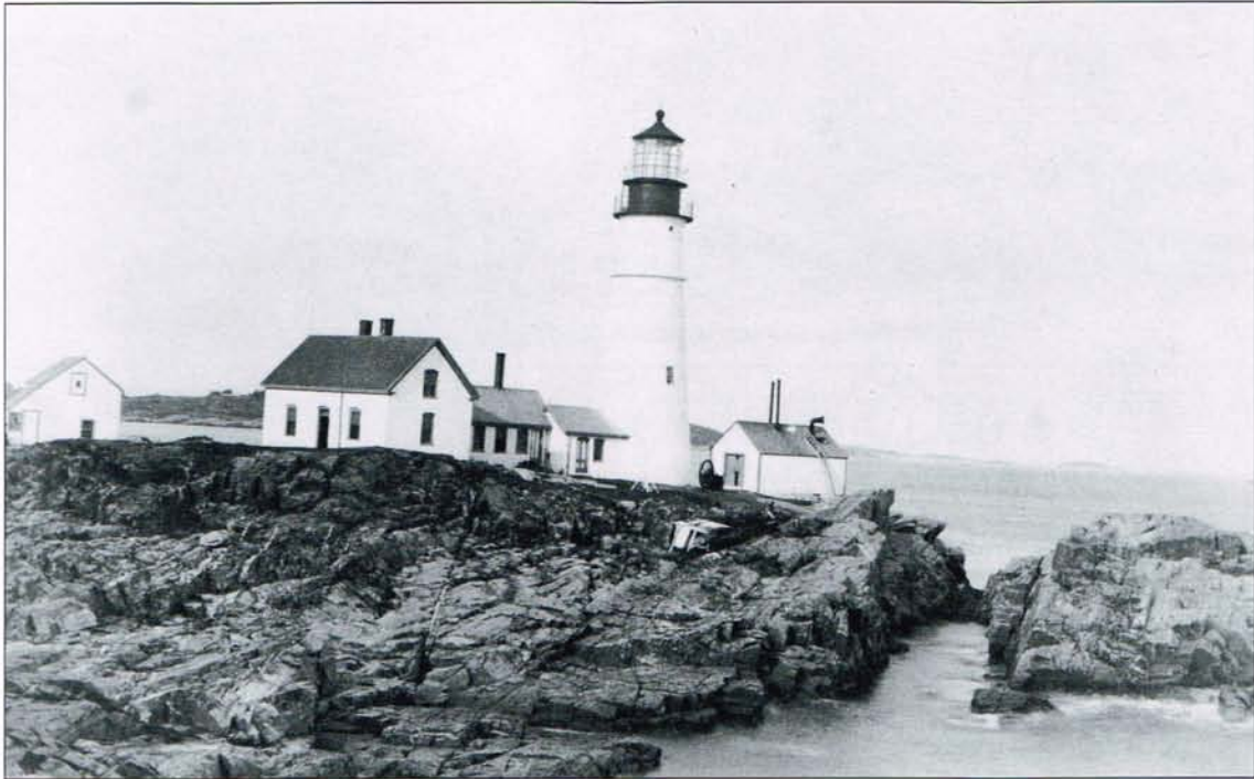
Above - This photograph, taken between 1887 and 1891, shows the brick fog signal house (at right) constructed to house the caloric engine transferred from the Boston station. The horn of the Daboll trumpet can be seen on the roof. The structure at far left is probably a barn. Photo courtesy of the Maine Historic Preservation Commission.
