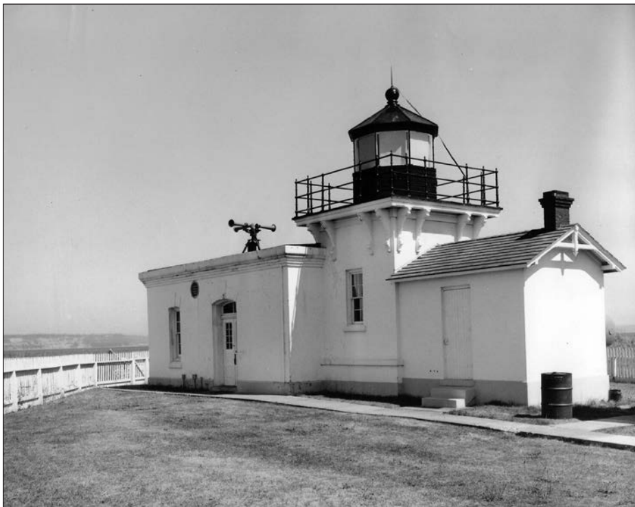
In 1953, when this picture was taken, Point No Point's fog signal had been upgraded from Daboll trumpets to triple diaphragm horns, seen on top of the fog signal building. Note the drapes drawn around the lens to protect it during the daytime. U.S. Coast Guard photo.
