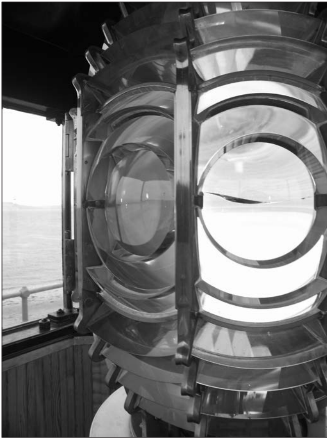
The crack in the bulls-eye of the Fresnel lens was caused by the fire in 1923. The lens is still in place in the lantern though not in use. Photo by the author.
