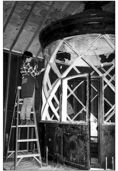
Above – Volunter Pam Hurst working on the badly deteriorated lantern room. Photo courtesy of PCLK.
