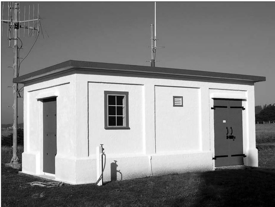
The oil house originally stored the kerosene oil for the lamps. It now contains the USCG VHF Repeater and Loran Monitoring Equipment. Note the antenna at left and on the roof. Photo courtesy of Bruce Rogerson.
