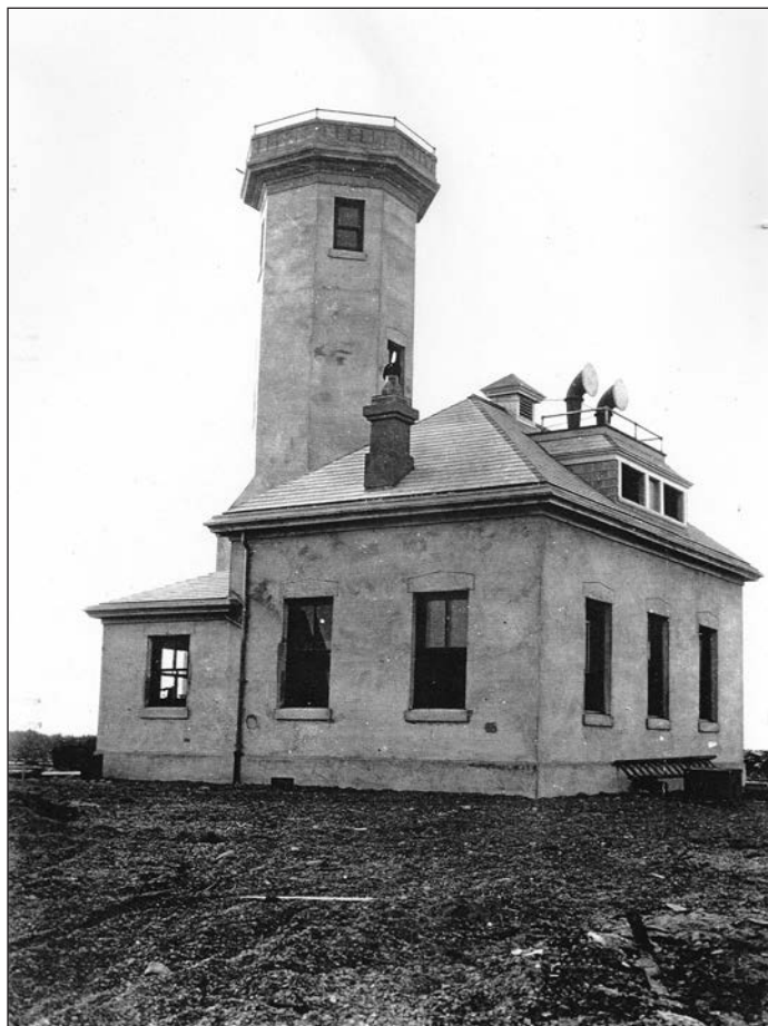
The new lighthouse under construction in 1913. USLHS archive photo.
