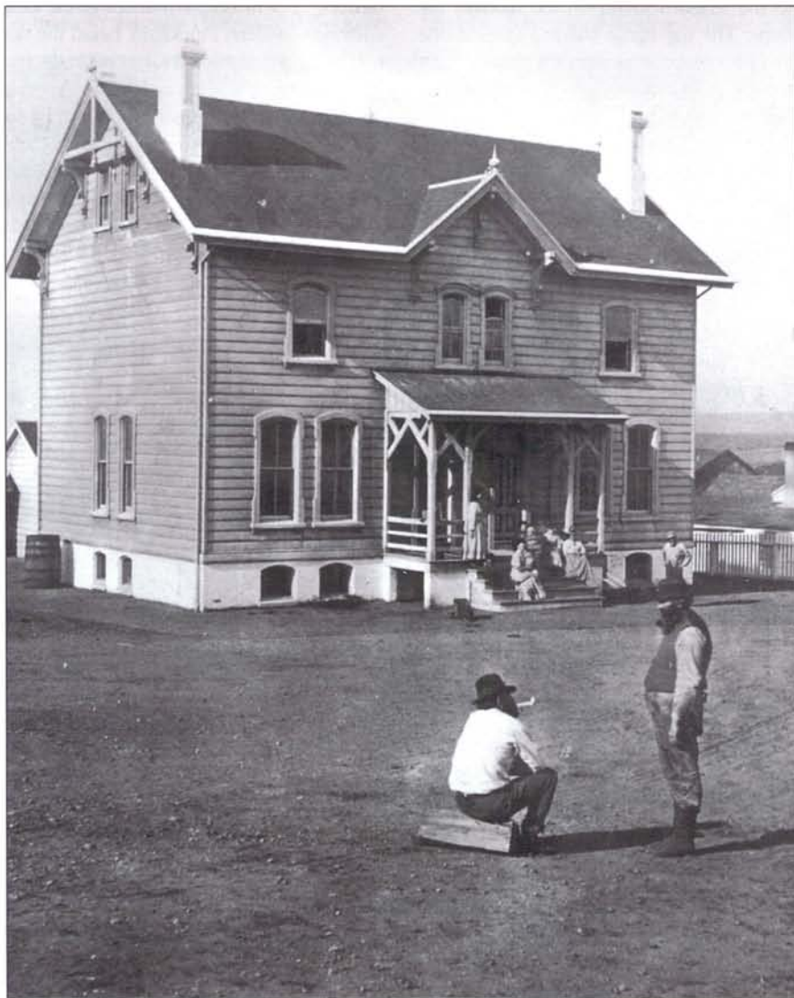
Keeper's four-plex dwelling shortly after completion. Photo by Eadweard Muybridge, courtesy of the Bancroft Library, U.C. Berkeley.
