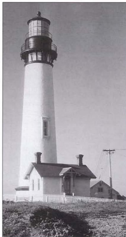
Above — Pigeon Point tower. The small structure at the base has an "office" and a room for lard oil storage. When the station started to use kerosene a separate oil house was constructed. USLHS photo circa 1930.
