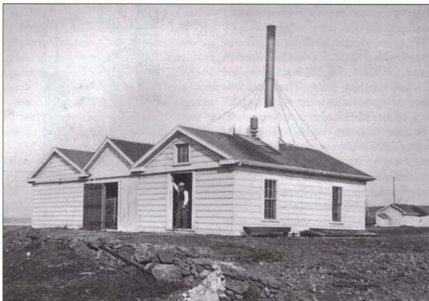
Below — The original fog signal building in the 1870's. Note the steam whistle fog signal in front of the baffle by the smoke stack. Bancroft Library photo.
