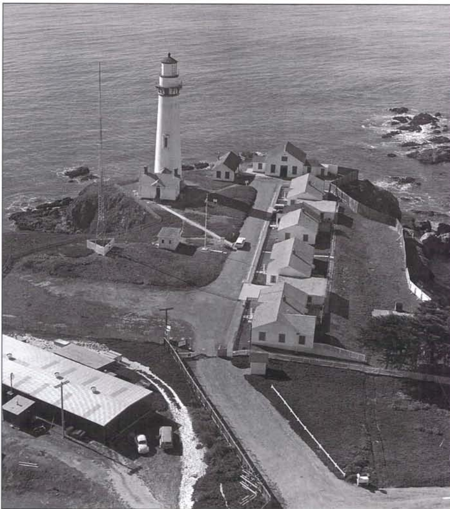
Pigeon Point station in 1970 showing the four ranch style dwellings which replaced the original four-plex. The fog signal is at the end of the driveway and paint shop/storage building to the left. The tall antenna was for the radiobeacon. The private structure at lower left has housed several enterprises, including an oyster farm. U.S. Coast Guard photo.
