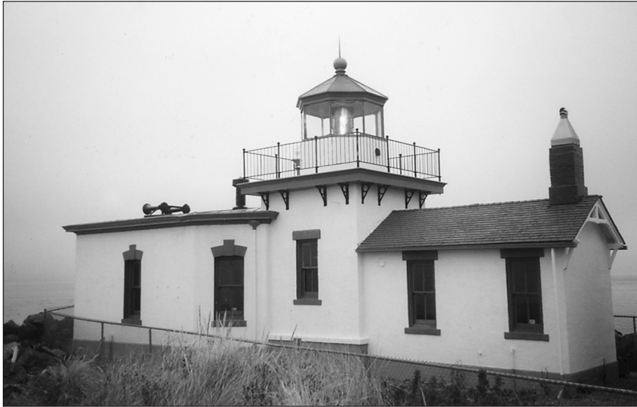
Above – Point No Point Lighthouse. Photographer unknown.
