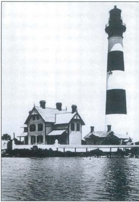
An 1893 view of the light station showing the water beginning to encroach on the grounds.
