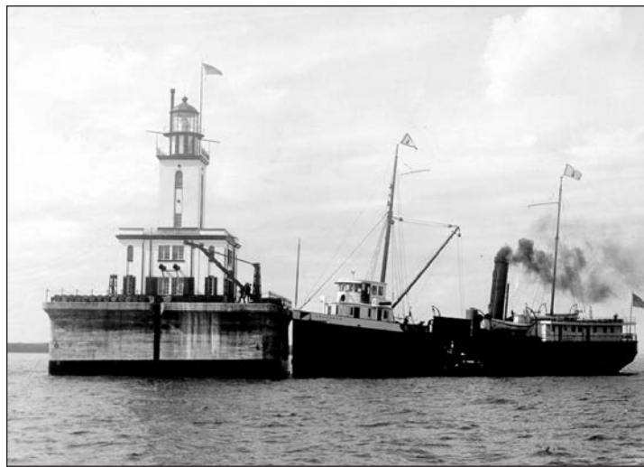
The lighthouse tender Amaranth alongside the Detour Reef Lighthouse in 1932. The first mast displays the U.S. Lighthouse Service flag, the second mast has the lighthouse inspector flag showing that there is an inspector onboard. U.S. Coast Guard photo.
