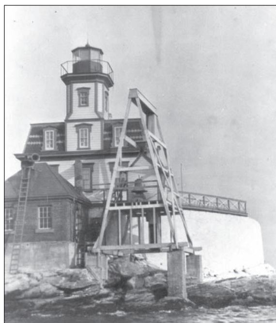
Left: The fog bell at Rose Island Lighthouse sits in a wooden frame. USLHS archive photo.
