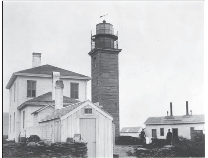
Beavertail Lighthouse was the site of many early fog signal experiments. In this photo the fog signal building, at right, has a whistle signal (in duplicate) installed. USLHS archive photo.
