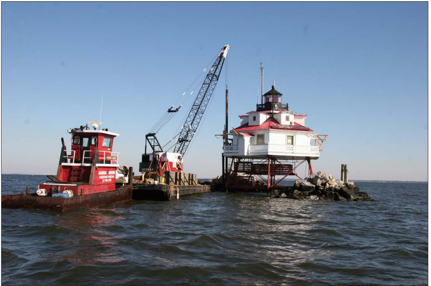
Driving the first piling for a dock at Thomas Point Shoal Lighthouse. Photo by Henry Gonzalez.
