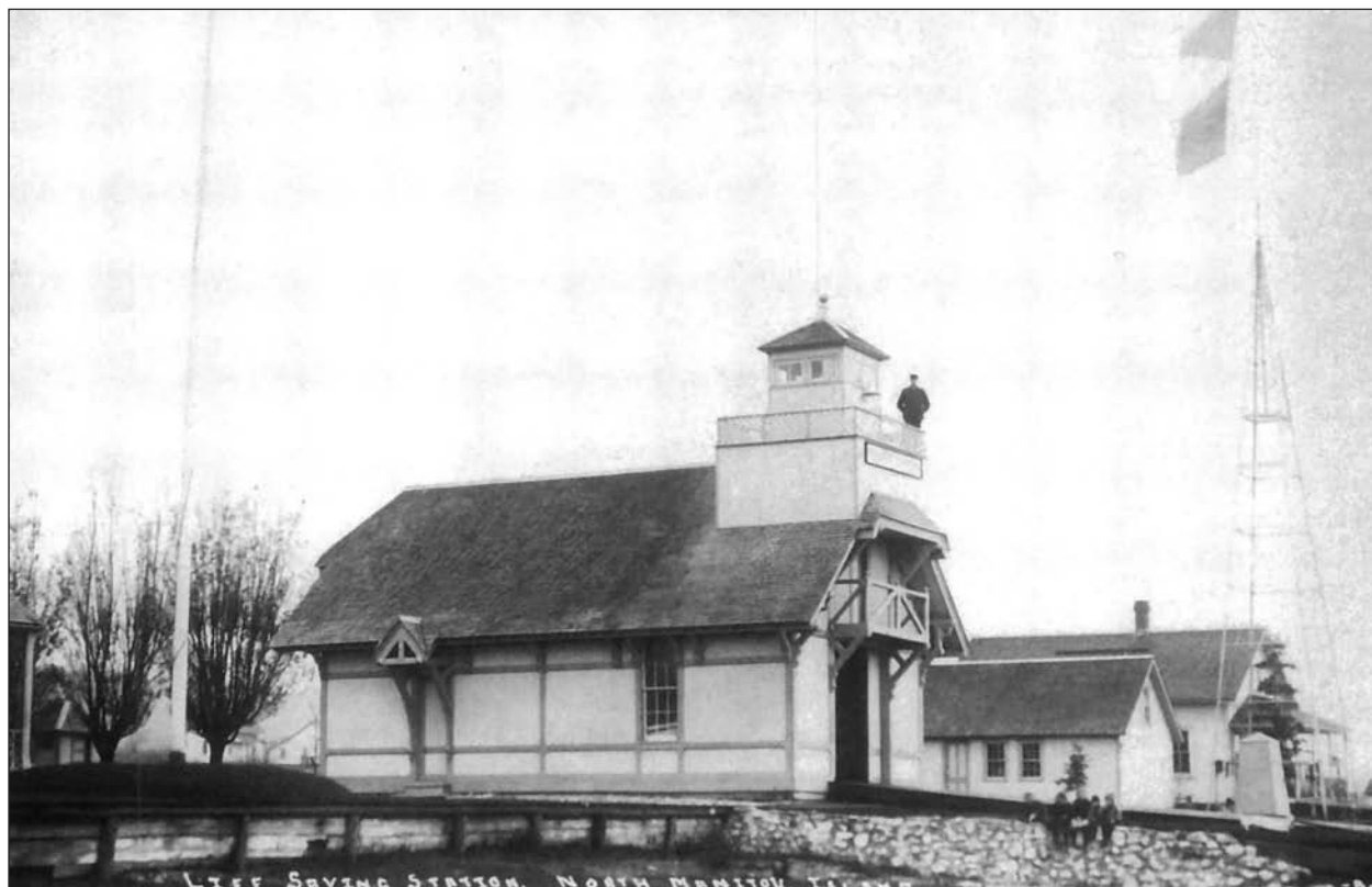
An 1880s design of a Life-Saving Service Station at north Manitou Island in Lake Michigan. Early station designs had an open platform for the watch stander. In this design, the watch room is enclosed. Note the watchman on the balcony and the small children in front of the marine railway. USLHS archive photo.
