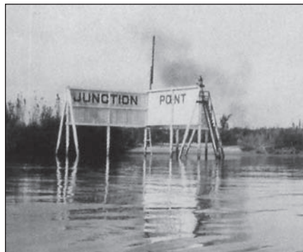
The Junction Point echo board in California's Sacramento Delta. USLHS archive photo.
