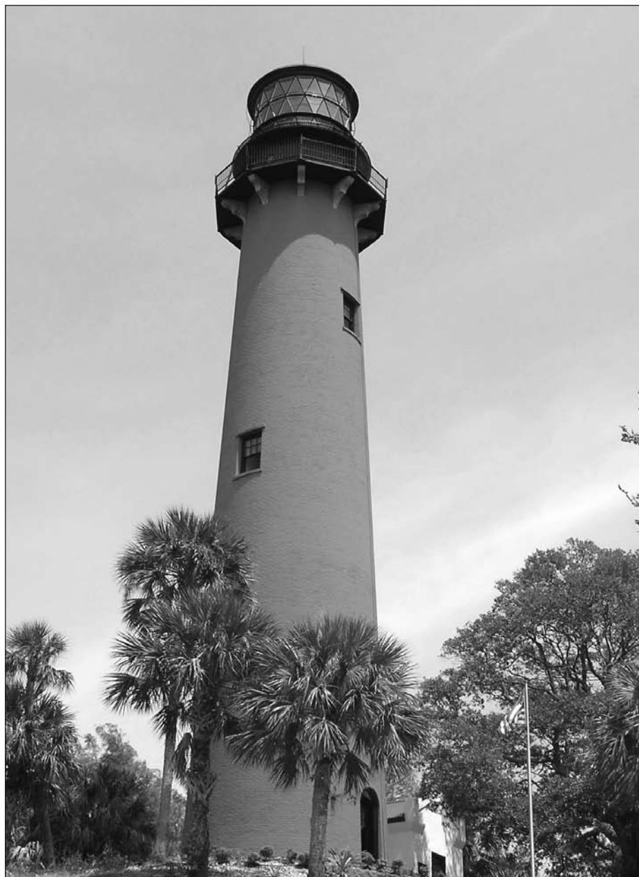
Jupiter Inlet Lighthouse as it is today. Photo courtesy of the Florida State Archives.
