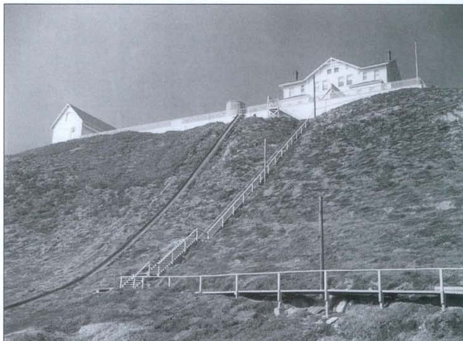
Supply chute from bluff to fog signal building at left, stairway at right. Photo by John Twohy.
