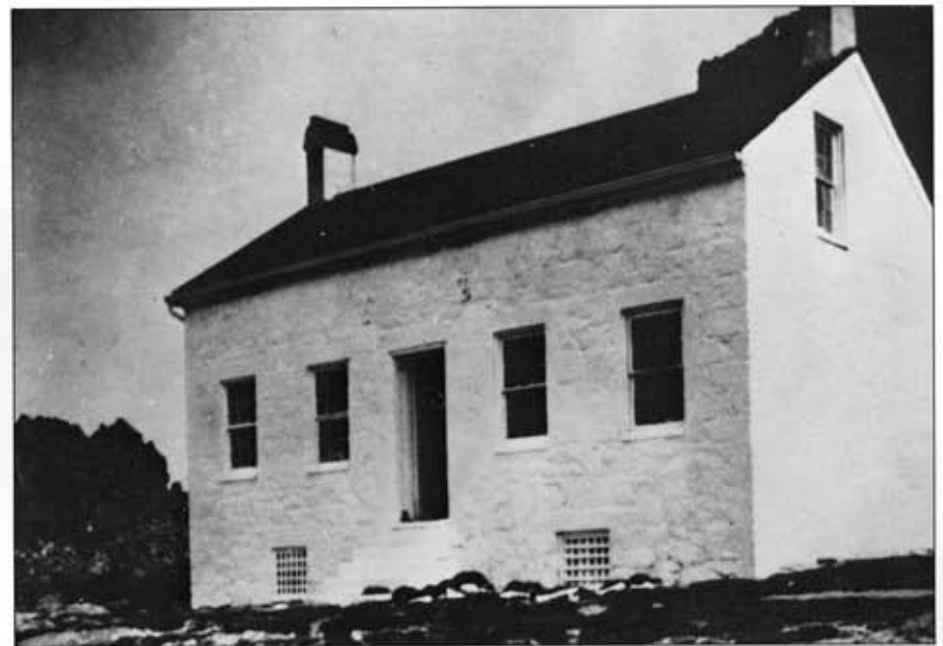
This 1 & 1/2 story stone house, containing only four rooms, was home to the keeper and his two assistants. All 16 of the lighthouses constructed on the west coast in the 1850's were of this design—13 had the tower incorporated into the house. This building was razed in 1969.
