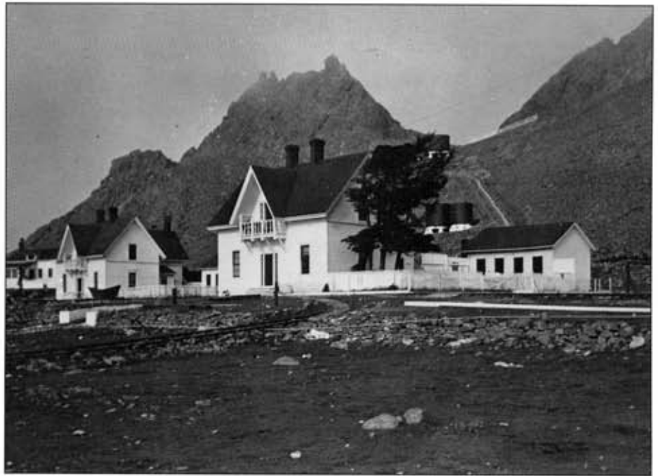
The addition of a steam powered fog signal in 1880 required more keepers and thus, the construction of these Victorian duplexes. The house on the left, presently used by U.S. Fish & Wildlife Service personnel, was constructed in 1878. The house on the right, now used by Coast Guard servicing personnel, was built in 1880. The original keepers' house can be seen at far left. Each family also had a small house (far right) which was used as a laundry and for storage. U.S. Coast Guard photo.
