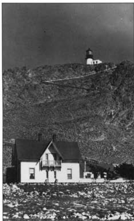
It's a long switch back hike from the keeper's house to the tower. The telephone type poles carried wires that linked the tower, fog signal building and all quarters with "call bells." USLHS photo.
