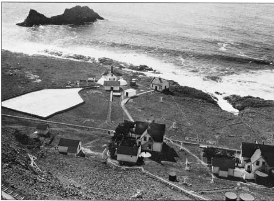
An overview of 'Farallon City' as seen from the hill. Water tanks are at the right foreground. The large white area at left is the rain catchment basin which directed water to the two cisterns located just in front of the fog signal building. The peaked roof building to the right of the fog signal structure was constructed circa 1910. It was used as storage and later as a fog signal building. U.S. Coast Guard photo.
