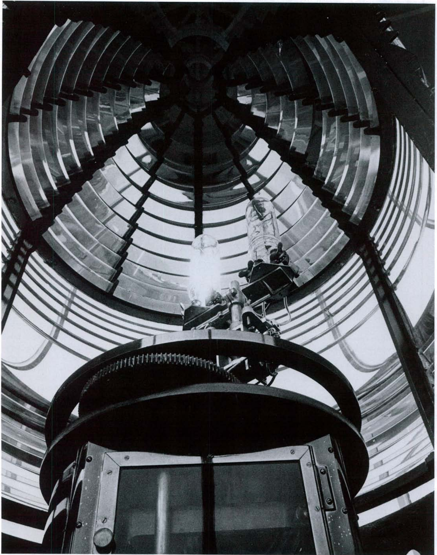
The original 3RD Order Fresnel lens that Emily Fish polished is still in operation. In later years a clockworks was installed that rotated a brass panel ("eclipser") which gave the light a flashing characteristic.
