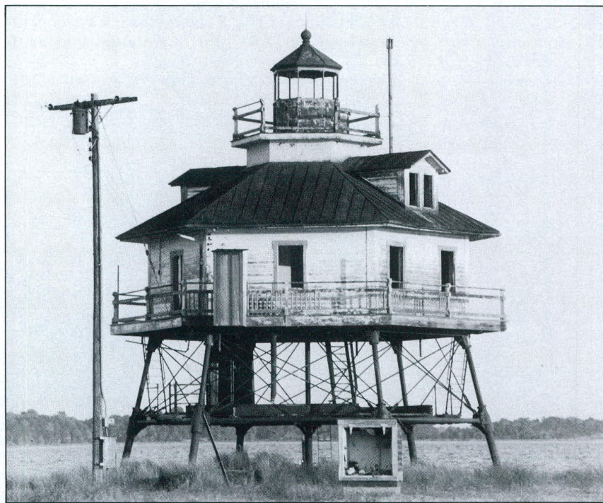
Drum Point Lighthouse circa 1950. Note electric lines running to the structure. The lighthouse is now high and dry at low tide and easy prey for vandals. Photo courtesy Calvert Marine Museum.
