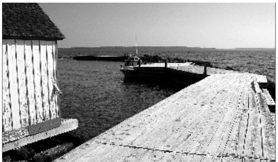
Below – The Devils Island boat house and landing at the south end of the island in 2001. Photo courtesy of Bob Mackreth.
