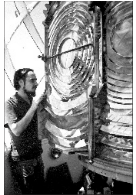
Above – A member of the Coast Guard working on the re-installation of the Third Order Fresnel lens in the Devils Island lantern, spring of 1976, photo by a local outfitter.
