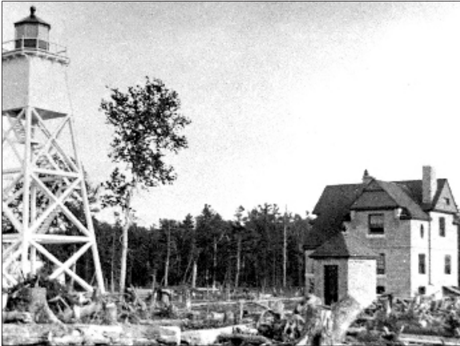
The temporary timber tower erected on Devils Island in 1891 while funding was being sought for the construction of the permanent cast iron and steel structure. National Park Service Collection.
