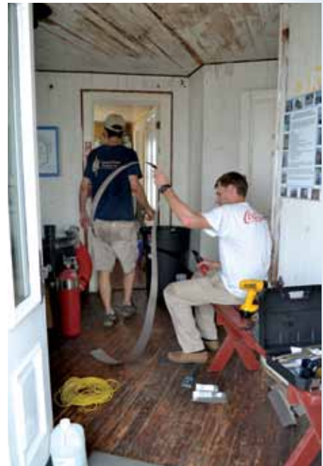
CLOCKWISE FROM TOP: Henry Gonzalez and the actual Thomas Point light; Craig Swift (left) and Leslie Morris from Keast & Hood, Co. working in the entry room; and Hobie Statzer (left) and Tony Pasek collaborating on a sanding project.
