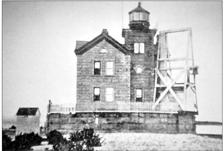
Cedar Island Light Station before 1910 with original fog bell tower. The open A-frame provided height for the falling weight to power the bell striker. U. S. Lighthouse Society photo.
