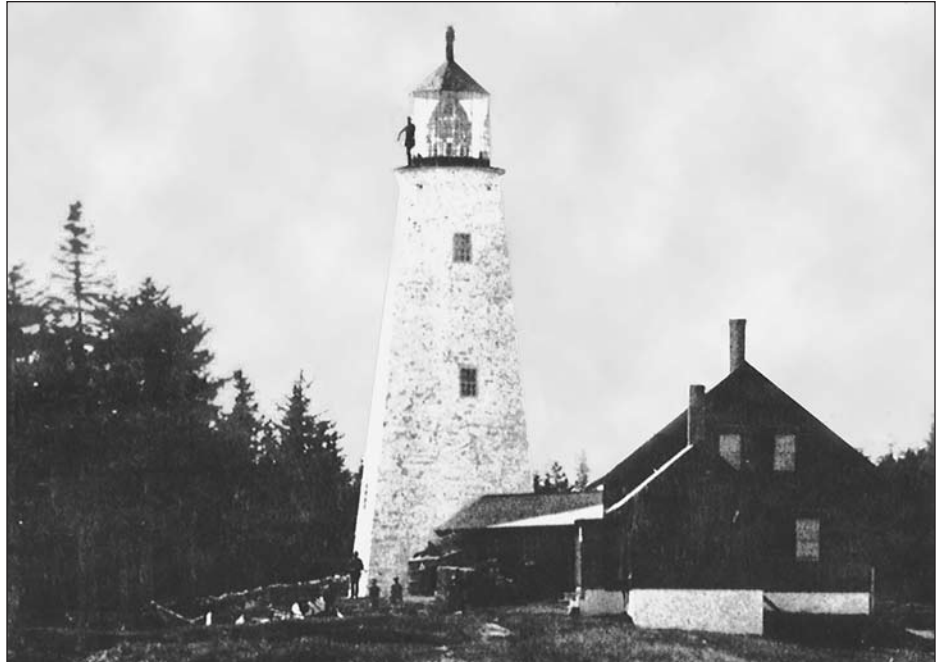
Above – Original rubble-stone octagonal Cape Elizabeth west tower. Note the Fresnel lens, keeper on the gallery and the other people (keepers' families?) gathered around the base of the tower. Photo courtesy of American Lighthouse Foundation.
