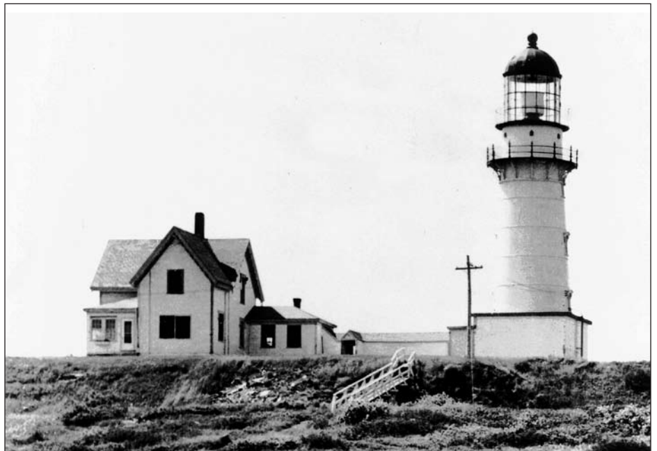
The 1873 cast iron east tower which is still in use today. Note the covered passage between the tower and dwelling. The power line pole indicates that the lamp is electrified. The Second Order Fresnel lens is shrouded in a linen cover. Photo Courtesy of Robert J. Lewis.
