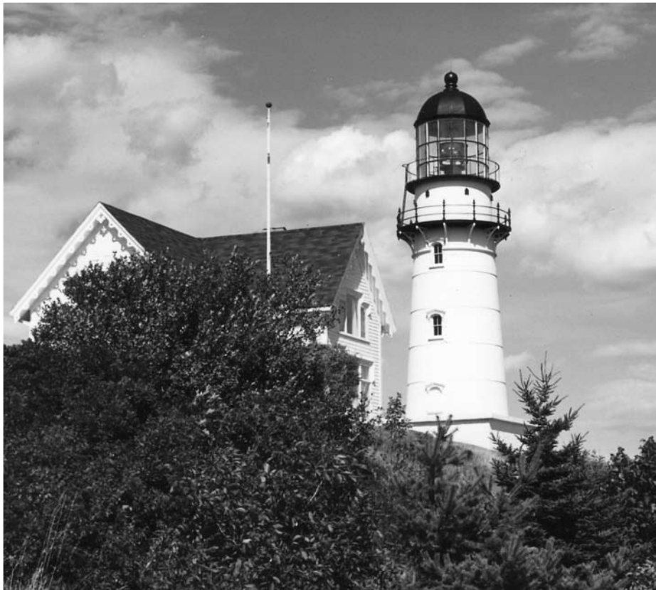
Above – East Tower showing the Second Order Fresnel in the lantern. This lens never had the top and bottom sections to complete the “beehive” shape. Photo courtesy of the Shanklins. Below – The Cape Elizabeth east tower Second Order Fresnel lens on display in the Cape Elizabeth town hall. The original characteristic of this lens was six rapid flashes followed by an eclipse of 17 seconds. Photo courtesy of Rusty Nelson.
