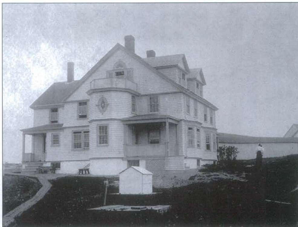
Below - The assistants' duplex dwelling after its "colonial revival" style renovations and before the covered walkway between the house and the tower was removed in 1900. The connecting walkway can be seen at right behind a keeper's wife checking her garden. National Archives photo courtesy of Sally Snowman.
