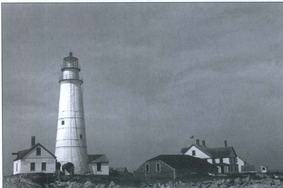
Fog signal horns can be seen on the roof of the building at left. Note the lines extending down the tower and scaffolding at the base. The keepers were responsible for painting the tower both inside and out. They pulled the scaffolding up to the lower walkway and lowered themselves as they painted. No extra pay was given for this yearly chore. U.S. Lighthouse Society photo.
