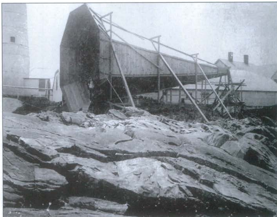
Above - The very large Daboll trumpet horn which measured 55 feet long and was 17 feet wide across the mouth. This horn was part of a 1864 experiment by MIT students. If you look closely you can see a person standing in the mouth. To the right of the horn you can see a portion of the duplex prior to the 1895 renovations. National Archives photo courtesy of Sally Snowman.
