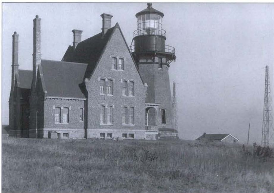
Block Island SE Lighthouse and dwelling circa 1948. Fog signal building roof in background. The two towers supported the radio beacon antenna. Note how tall the duplex dwelling chimneys are. They were reduced in later years. U. S. Lighthouse Society photo.
