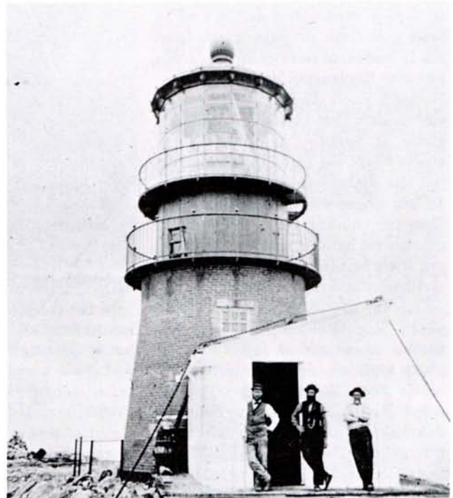
Above: Workmen standing in front of the Farallon Island tower circa 1856. The first tower was too small to accommodate the 1st Order lens.
