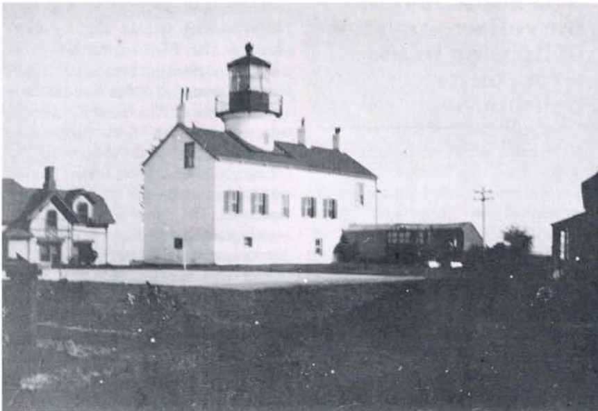
Alcatraz Lighthouse—1908 just prior to demolition. Note the cellar is above ground and that this structure did not receive the leanto kitchen addition added to the other seven.
